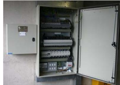
In all there were 52 sensors, 10 receivers and 10 **Oracle II** controllers fitted to the car parks allowing each floor to be split into two levels.
